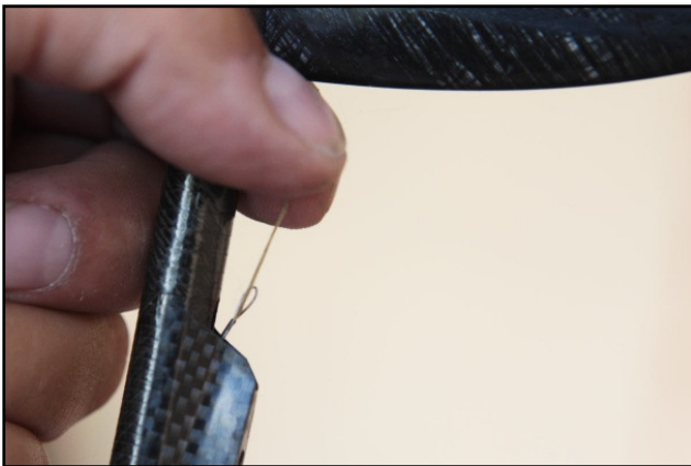
Figure 2.13-The thread on the cable of the elevator
