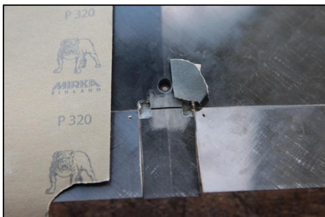
Fig. 2.18 – preparing axle bond with sandpaper
